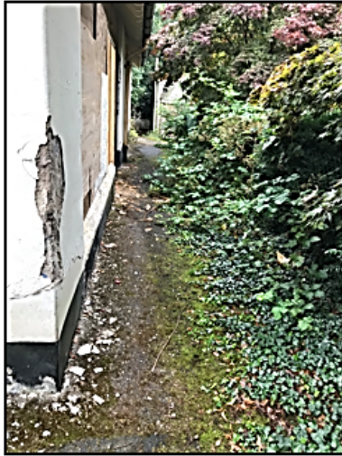
Building 02, damaged render to be repaired,
